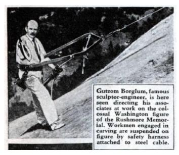
"There are no reserved seats at Rush-more. Workmen when engaged in actual carving are suspended over the edge of the cliff in steel and leather harnesses attached to a 3/8 inch steel cable. These cables are 'paid out' or reeled in by hand winches.
