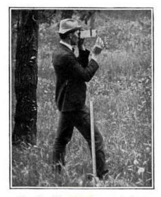
FIG. 65.—The mirror hypsometer in use.
